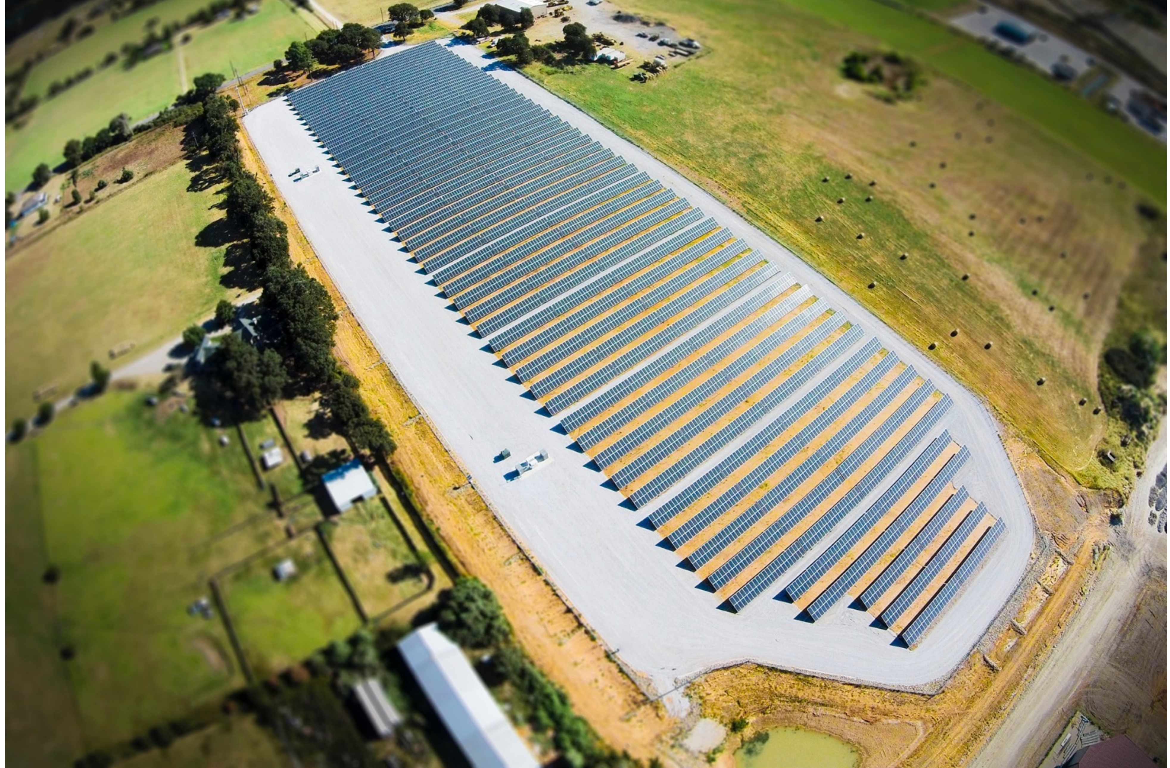
Solar array, Georgia
