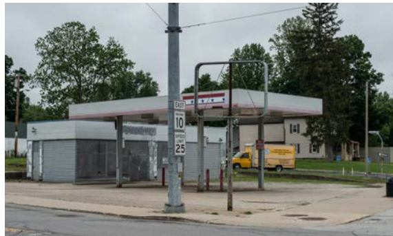
The Town has been pursuing the old Speedway site to potentially redevelop this site as a public common area.
