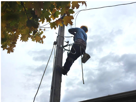
Lineman repairing overhead utility line.
